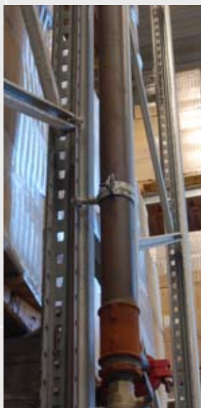
Integrated sprinkler system
