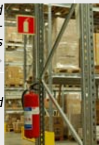
Integrated fire extinguishers
